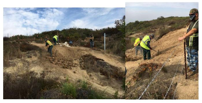
Breaking up large bike jump area. Workers pulled out over a dozen bags of dirt that formed the jump. Ground was left loose, broken up and dead brush was placed in the area. Site was monitored by Native American and archaeological contractors due to the proximity to sensitive resources. No cultural resources were detected.
