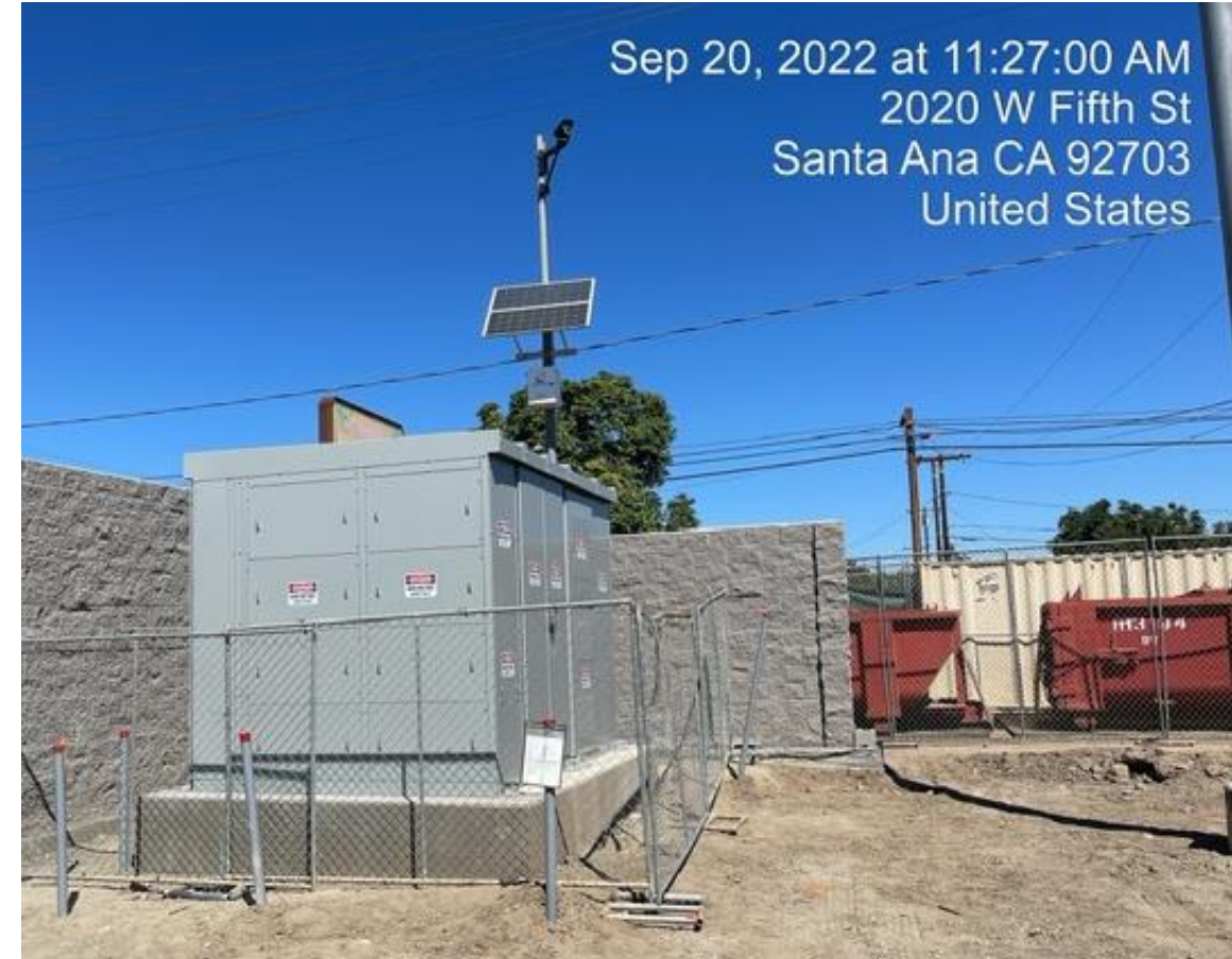
Southern California Edison (SCE) metering switchgear
