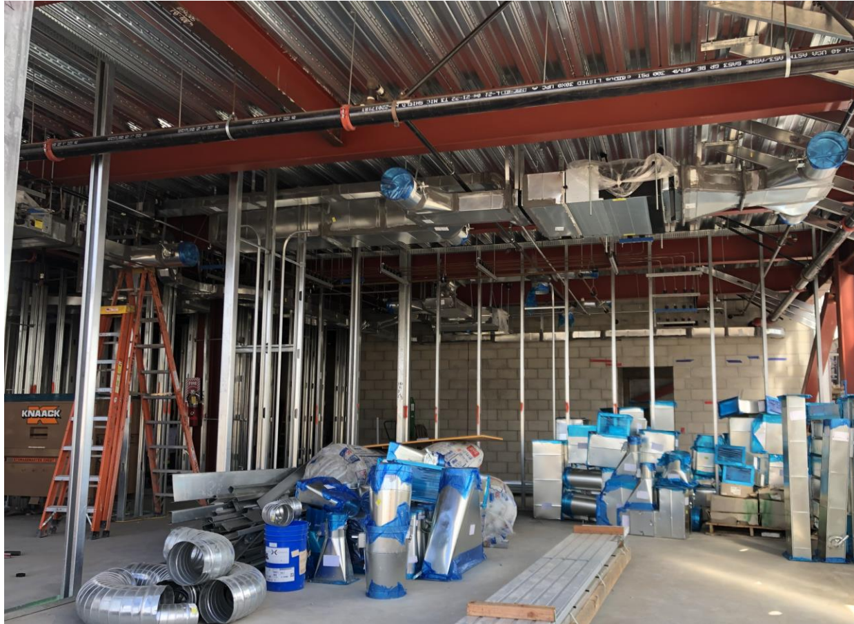
Interior walls, piping and heating, ventilation, and air conditioning
