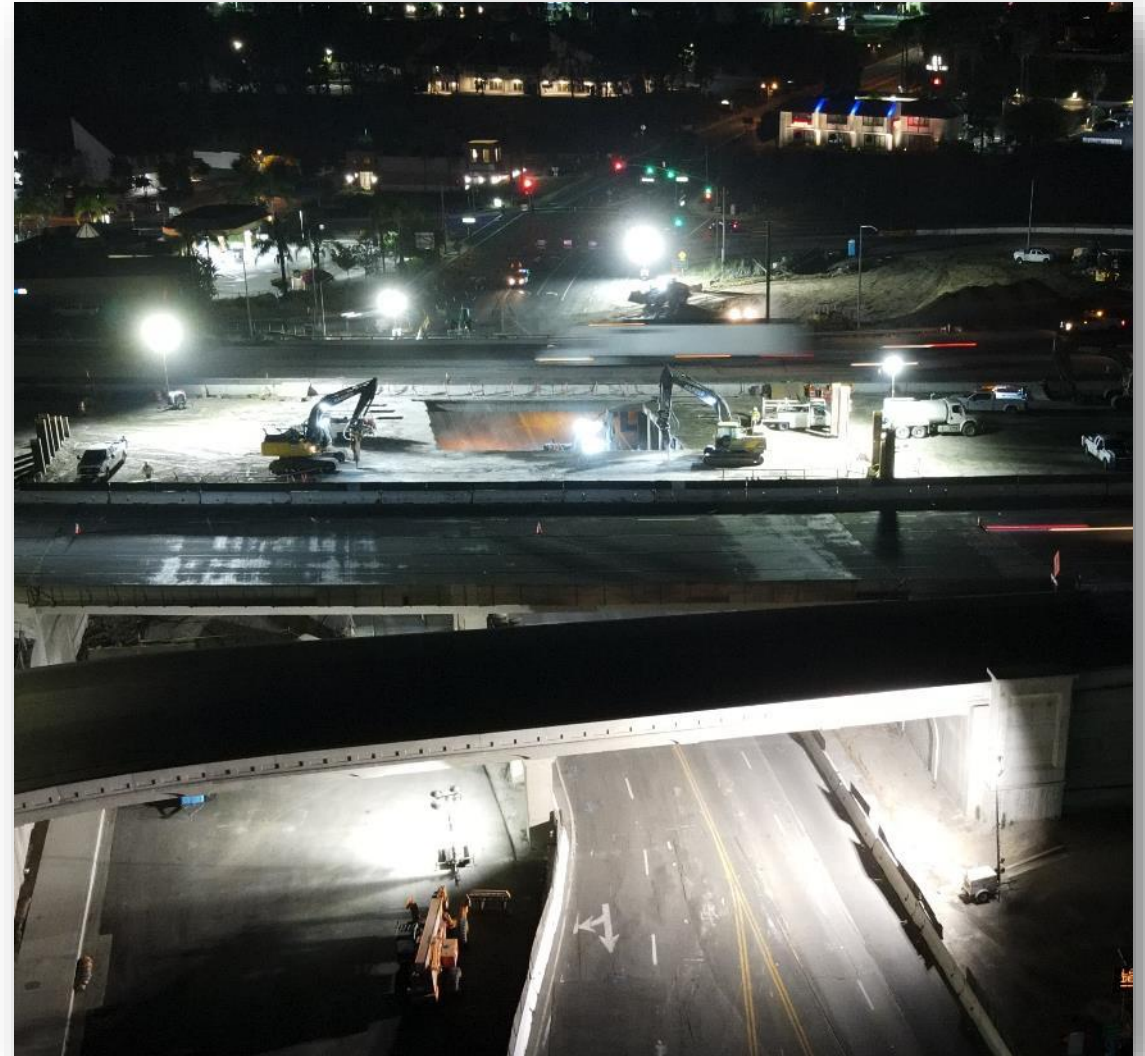
Bridge demolition at La Paz Road
