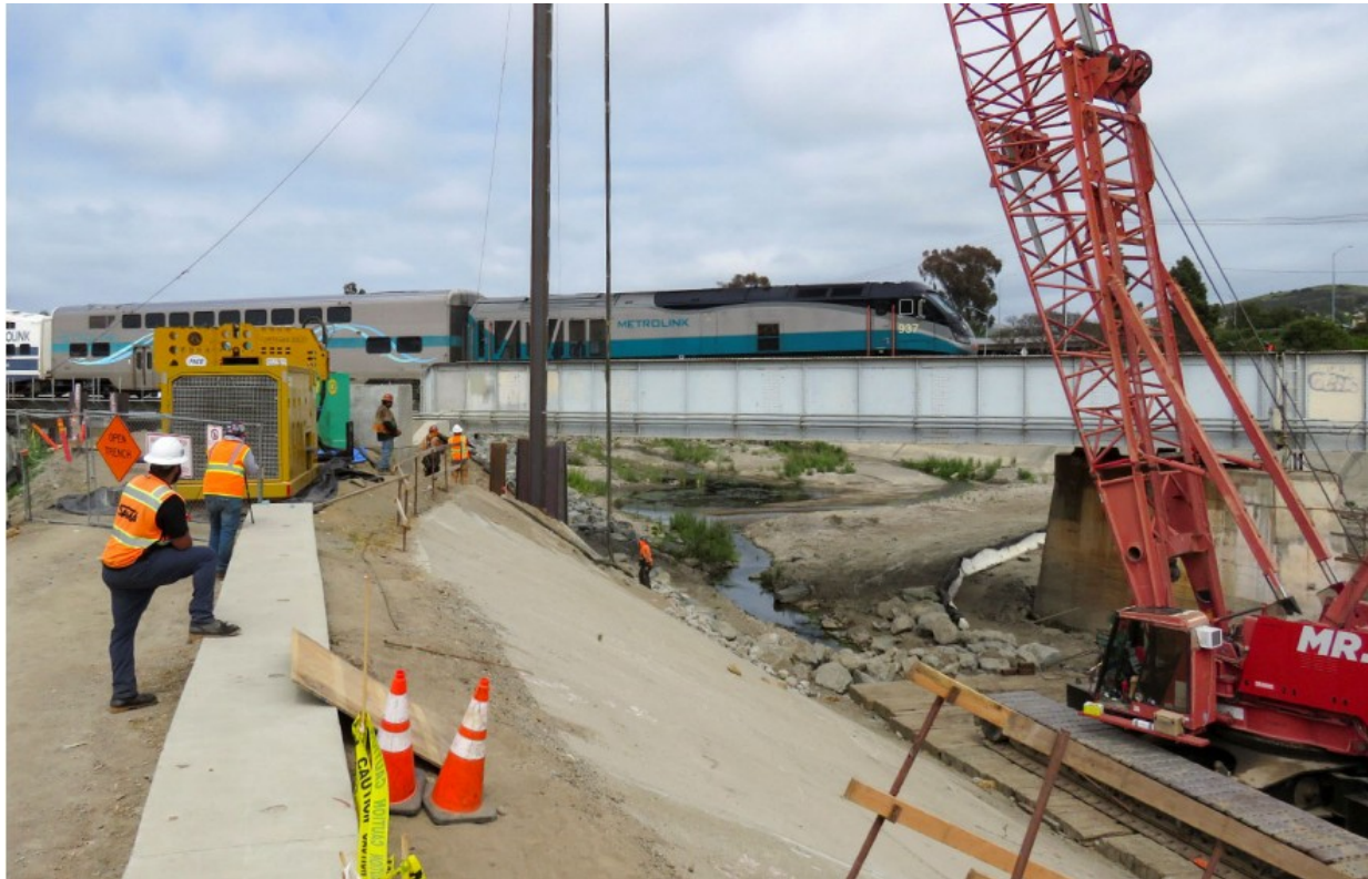
Contractors installing sheet pile walls
