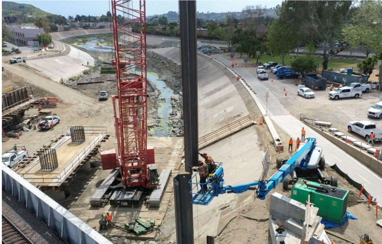
Contractors installing sheet pile walls
