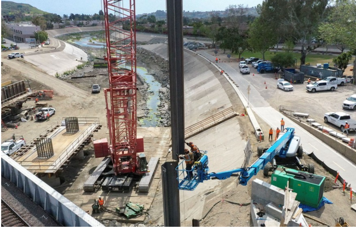
Contractors installing sheet pile walls.
