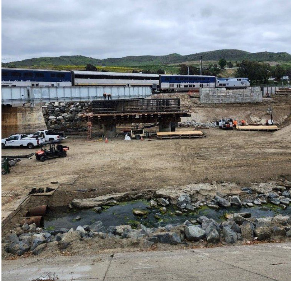
Diversion channel redirecting water flow around the construction site.
