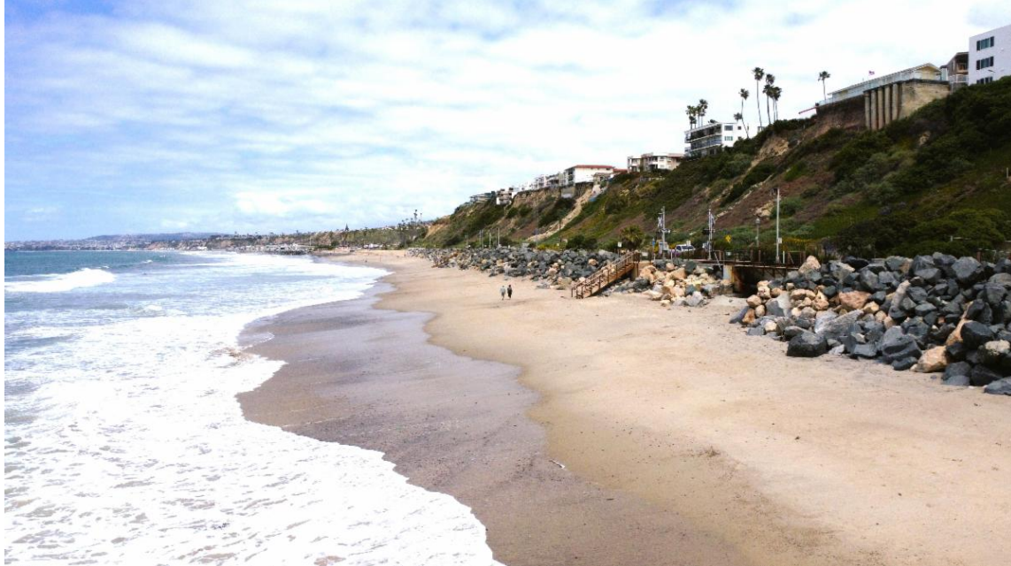
Before Photo: Riprap conditions near Dije Court beach access
