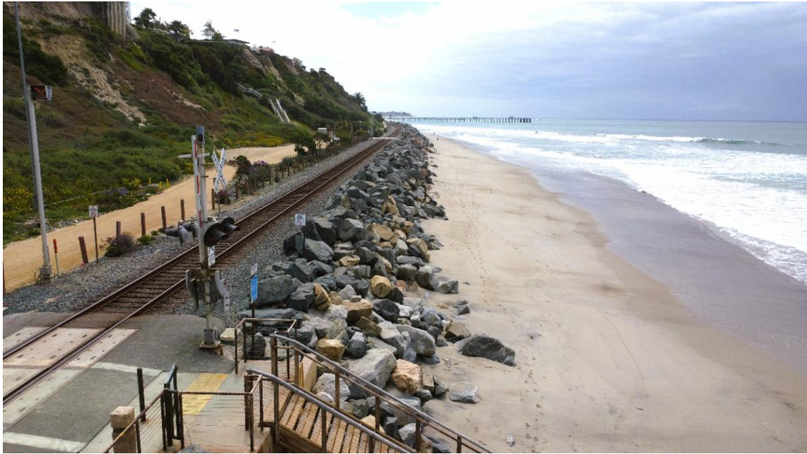
Before Photo: Riprap conditions near El Portal beach access
