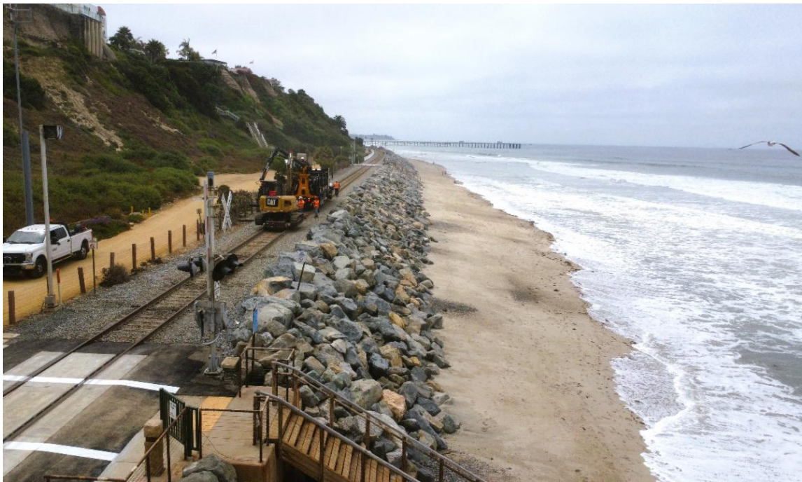
After Photo: Final riprap conditions near El Portal beach access
