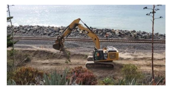
That work will involve drilling large steel anchors more than 100 feet long into the bedrock of the slope adjacent to the railroad track to prevent it from pushing the track further toward the ocean. The track moved as much as 28 inches between September 2021 and September 2022 due to storm surge and sand erosion on the coastal side and the gradually sliding hillside on the other.
