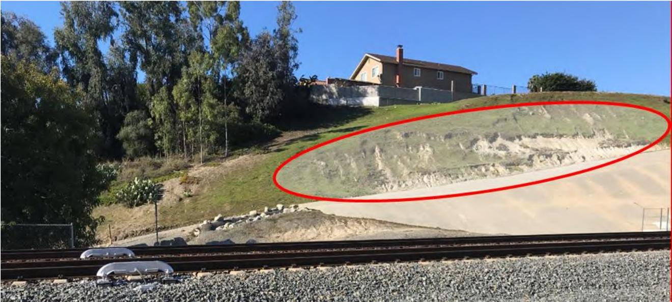
Cut slopes at a 2H:1V inclination in this material are likely grossly stable. Most of the west side cut slope has established shallow root vegetation consisting of grass and ice plant. However, the denuded west side slopes have erosion rills and upwardly progressing shallow arcuate scarps generated from surficial sloughing. A perched or shallow groundwater condition is not anticipated at the site. The soils at the site may have dispersive properties.
