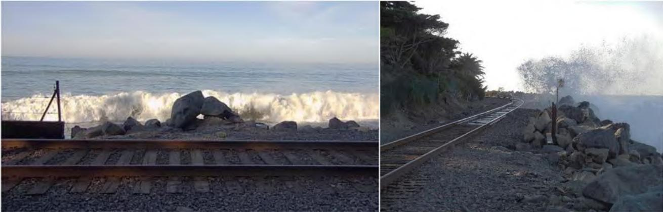
Portions of the southern coastal corridor are protected by rip-rap revetment. These areas include MP 203.85-204.53, 205.15-205.42, 205.88-206.21, and 206.9-207.2 (Figure 14). Some other portions of the rail are protected by rock with soil and vegetation.
