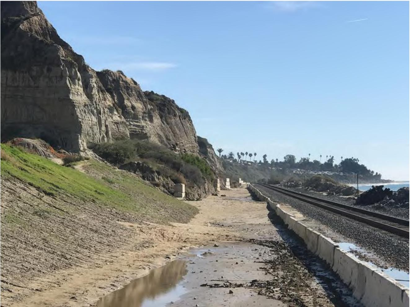
The hillside erosion and discharge of water and sediment under the rail can provide sediment to the beach. If the eroded sediments are collected and hauled offsite or left in place on the landward side of the tracks, this can deprive one of the historic supplies of sediment to the beach and may contribute to the ongoing erosion and loss of beach along this coastline.
