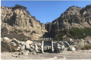
At San Clemente State beach, there are stacked concrete Interblock units placed at the mouth of finger canyons to slow sediment transport. Very heavy accumulations of sediment are being blocked by placed K-Rail (Figure 17).
