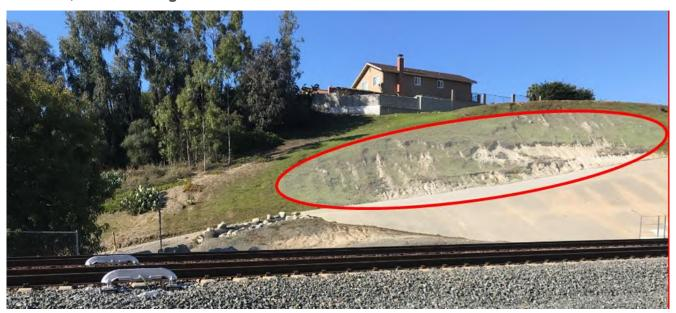
Cut slopes at a 2H:1V inclination in this material are likely grossly stable. Most of the west side cut slope has established shallow root vegetation consisting of grass and ice plant. However, the denuded west side slopes have erosion rills and upwardly progressing shallow arcuate scarps generated from surficial sloughing. A perched or shallow groundwater condition is not anticipated at the site. The soils at the site may have dispersive properties.
