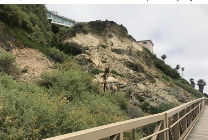
FIGURE 15 | Recent Landslide at MP 204.20 in contact with the Mariposa Walkway Bridge deck
