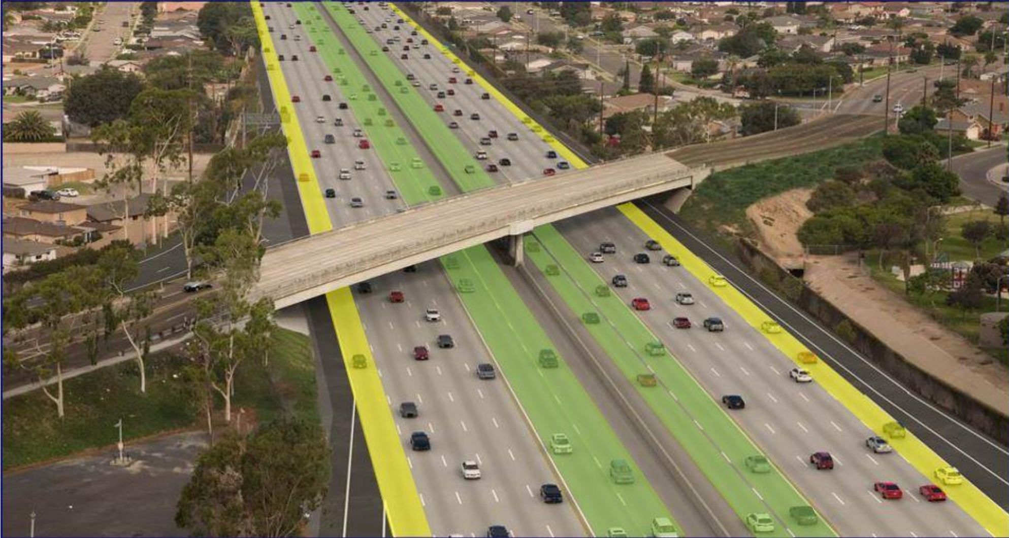
I-405 looking northwest at Springdale Street bridge
