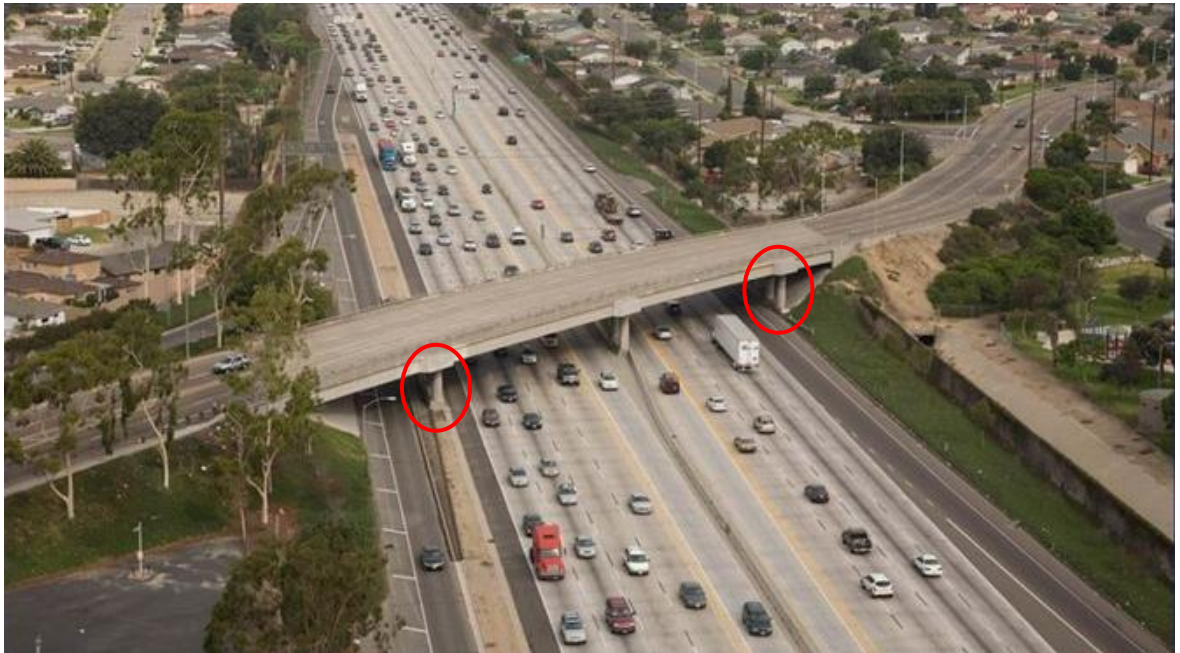
Existing I-405 at Springdale Street
