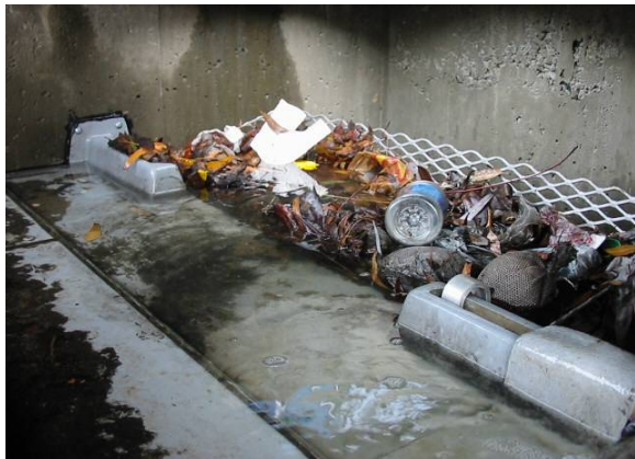
Curb Inlet Basket with Easy Maintenance Shelf System – 4' Wide Basin with One Wing
