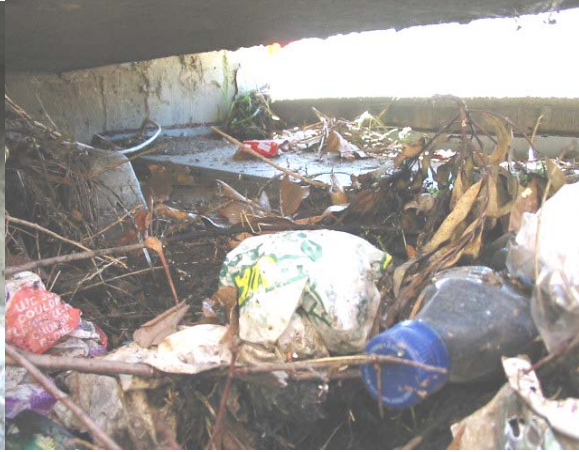
Accumulated Trash & Debris in Filter Basket and Shelf System LA County
