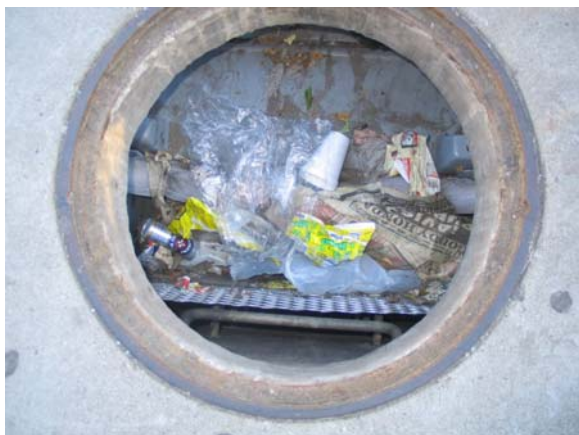
Curb Inlet Basket with Easy Maintenance Shelf System Positioned Under Manhole
