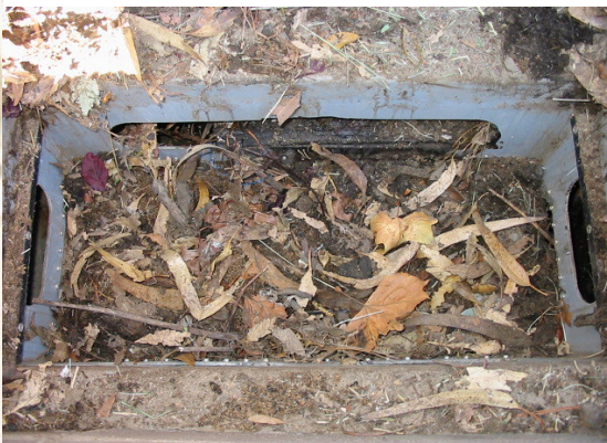
Grate Inlet Skimmer Box at Full Capacity. Bypass Prevents Flooding When Filter is Full Mission Avenue, Fallbrook CA
