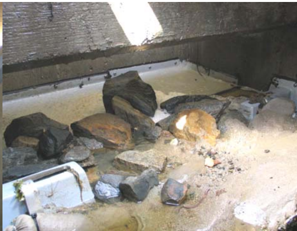
Hundreds of Pounds of Rocks and Sand Accumulated on the Curb Inlet Basket and Shelf System. This system can hold up to 500 pounds.
