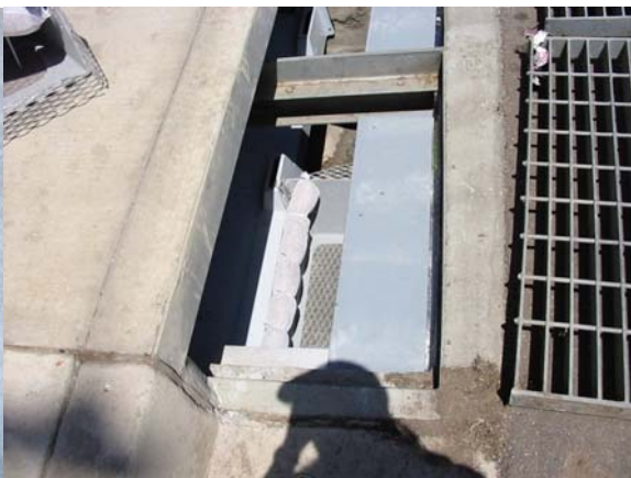
Curb Inlet Basket with Shelf System Installed in a Grate-Curb Combination Inlet
