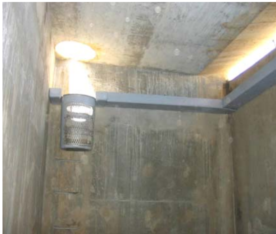
Custom Designed Shelf System with High Capacity Basket for a 30' Wide Catch Basin in City of Corona
