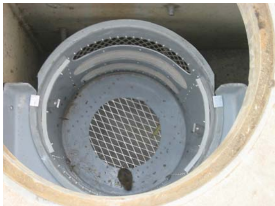
Curb Inlet Basket Positioned Under the Manhole for Easy Maintenance Poplar St. South of Birch, City of Brea
