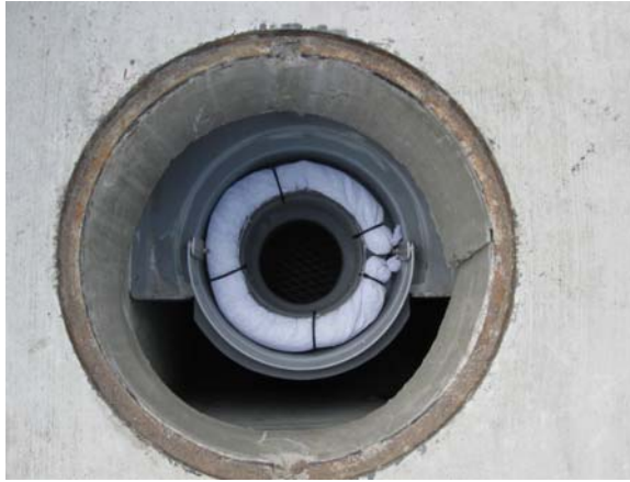
High Capacity Curb Inlet Basket Shelf System Positioned Under Manhole
