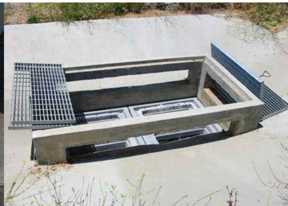
Customized Installation of 4 Grate Inlet Skimmer Boxes in a 4' by 8' Basin.
