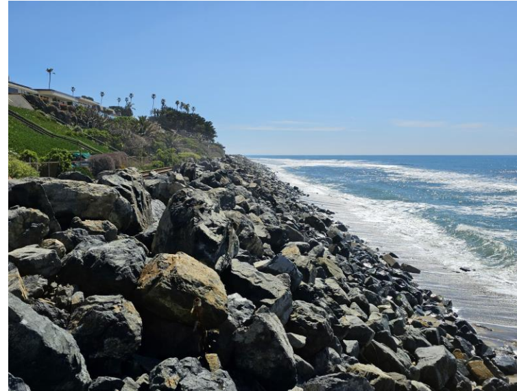
Monitoring Area #7 MP 206.70 – 207.25 Cyprus Shore to County Line
