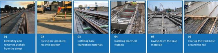
01 Excavating and removing asphalt from the street
