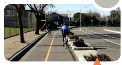
Provide a two-way Class IV Cycle-Track with buffer on the bike lane (OC Loop Gap L proposed alignment)
