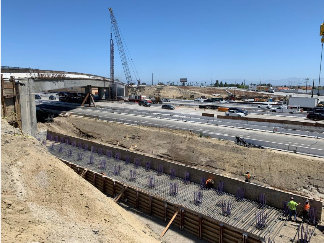
Goldenwest Street bridge construction
