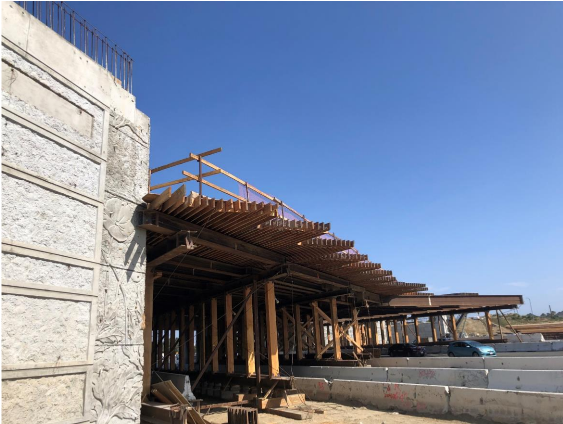
Brookhurst Street bridge construction
