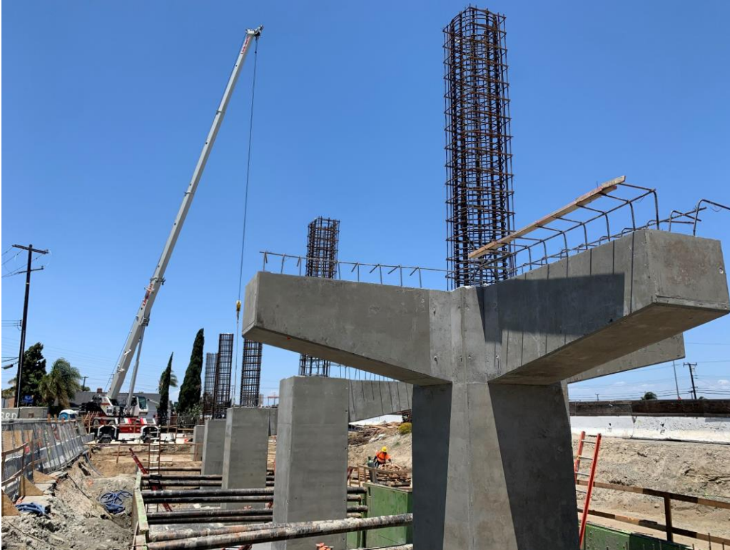
Heil Avenue pedestrian overcrossing construction
