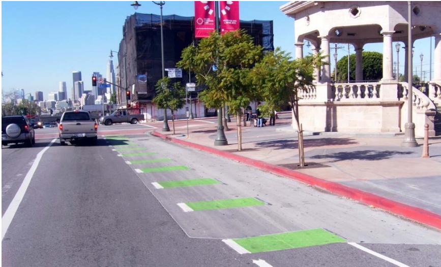
Green Paint at Conflict Points
