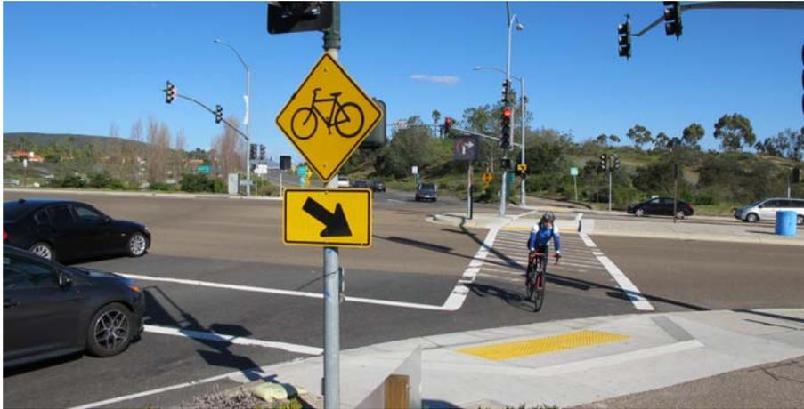
A cyclist from a bikeway, approaching an intersection with a local road and freeway ramps presses the crossing button and rides through on the lit pedestrian signal. Simultaneously, a no-right-turn-on-red arrow alerts drivers to wait for a green light.
