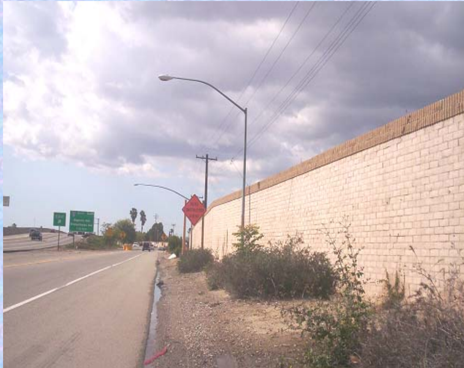
On-going construction SR-91
