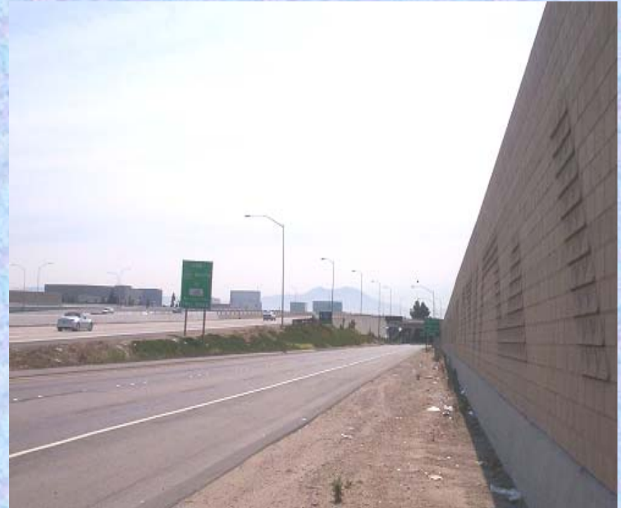
Unsafe work area I-405
