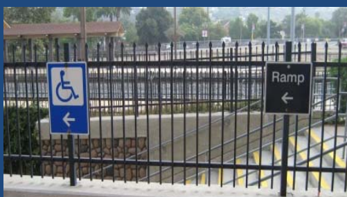
Old Town Station
