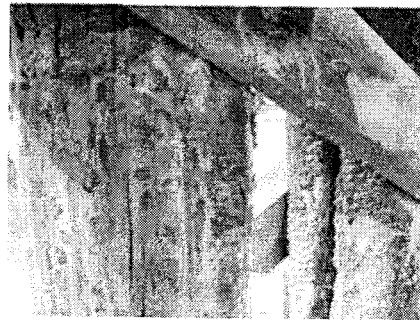
Pile "bent" showing past charring and cracking
