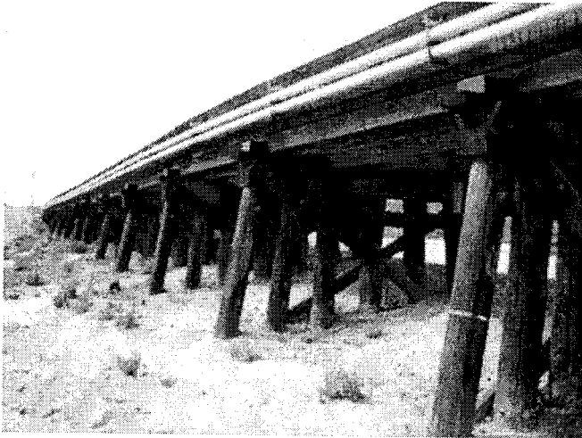
Bridge 207.6 North Approach.
