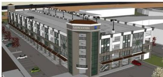
The five-level structure features energy efficient LED lighting, solar panels on the roof to power the facility and electronic signage at the entrance to display where parking spots are available.
