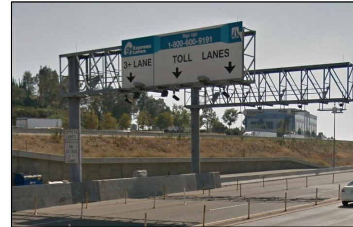
Existing WB 91 Express Lanes Toll Gantry
