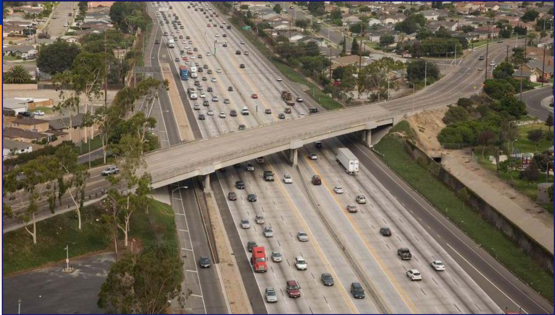
405 Freeway looking NW at Springdale St Overpass
