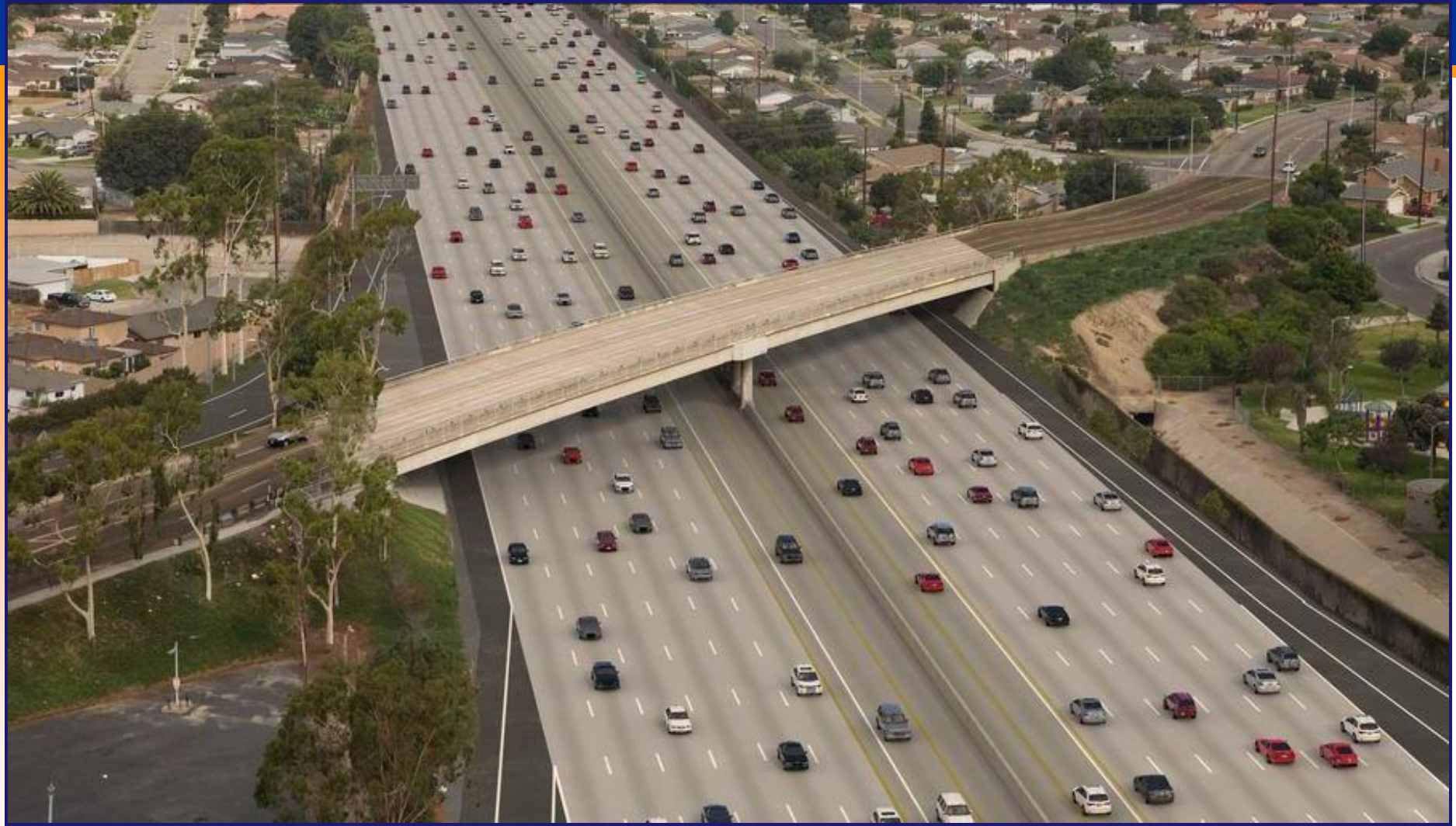
Two general purpose lanes added
