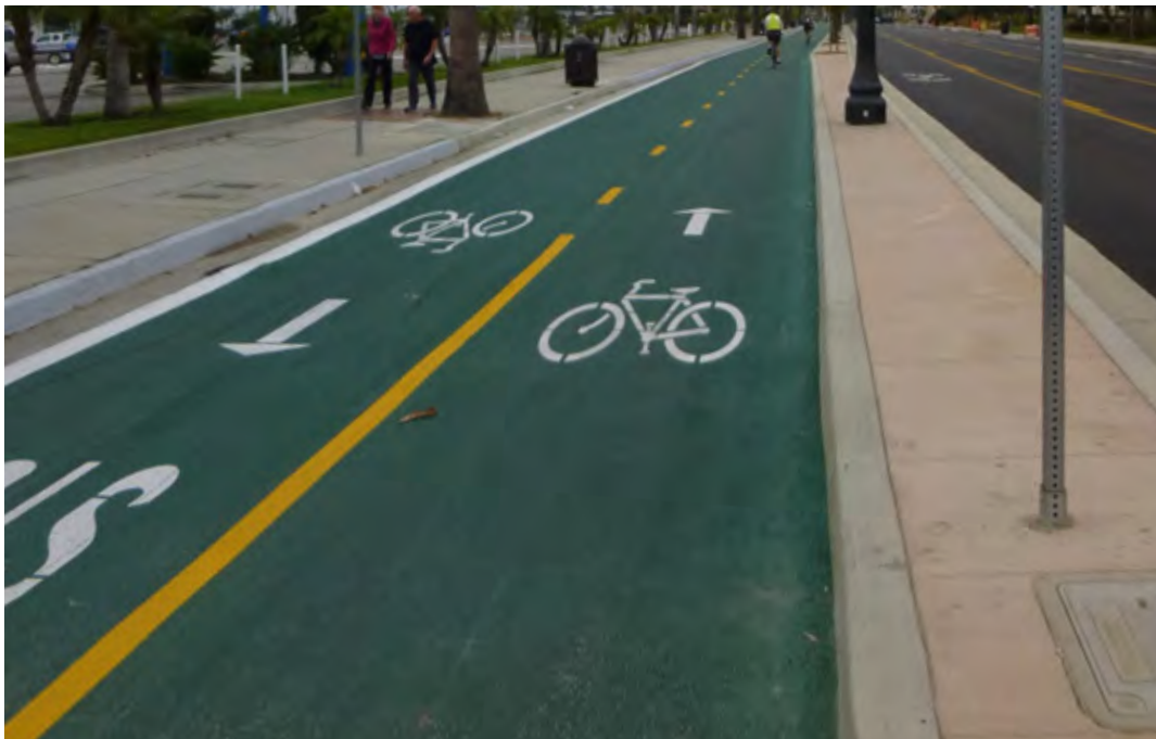
Two-Way Cycle Track (Separated Bikeway) Westwood Blvd, Redondo Beach (Photo: Jim Lyle)
