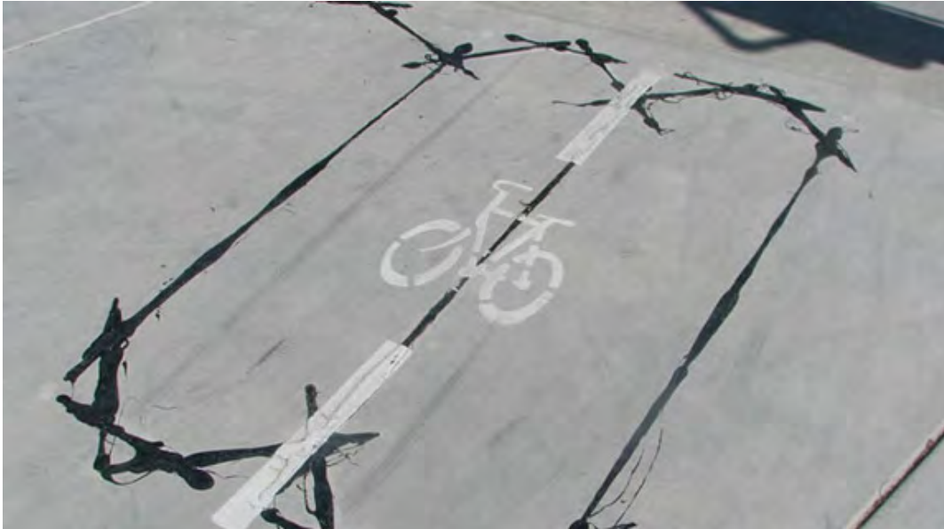
Bicycle Detector Pavement Marking, San Luis Obispo (Photo: NACTO)
