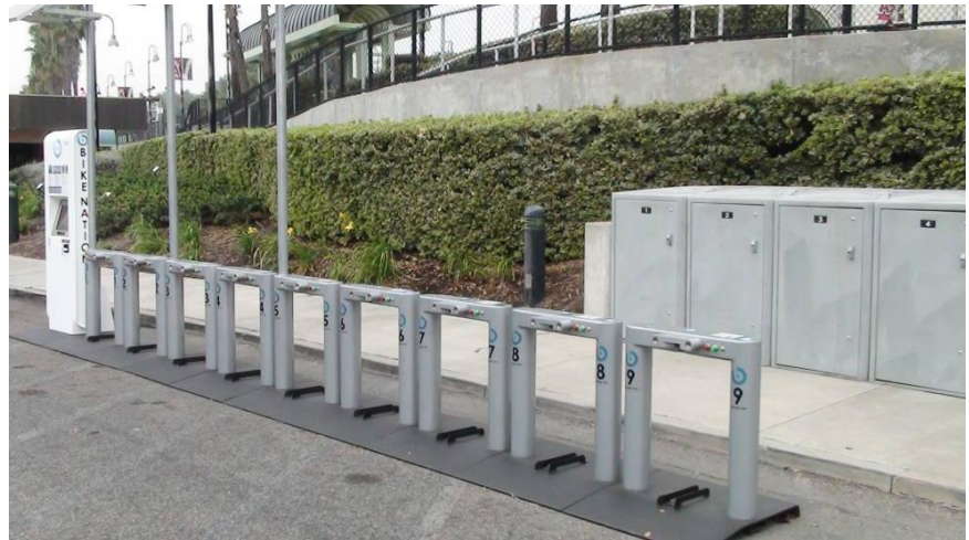
Bikeshare kiosk with bicycle lockers in background.
