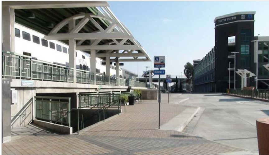
View of the station looking east.
