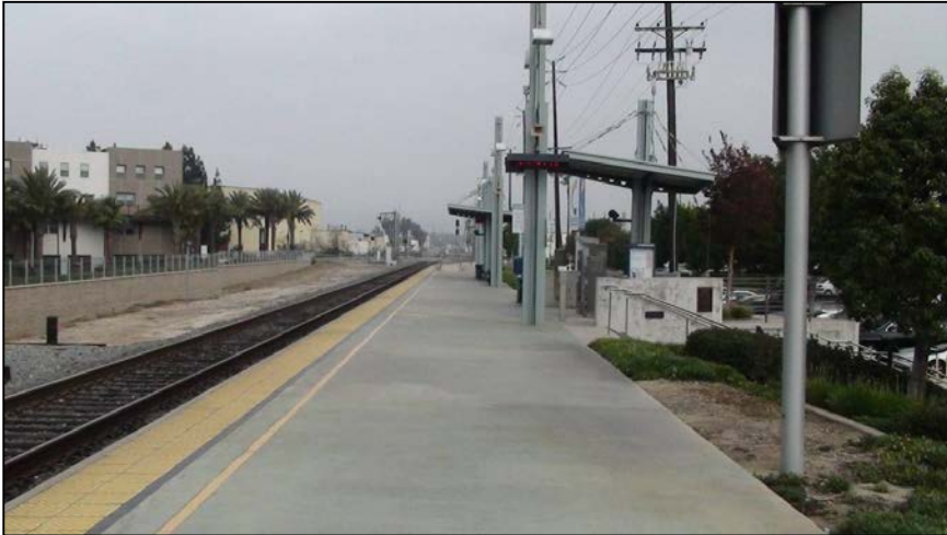
View looking north on the platform.
