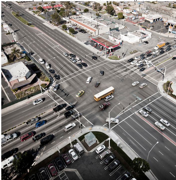
M2 funds help repair and rehabilitate the streets of Orange County.
