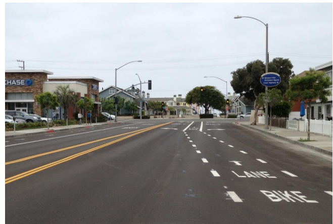
Image 1: Roadway reconfiguration to provide bicycle lanes. (Source: City of Newport Beach)
