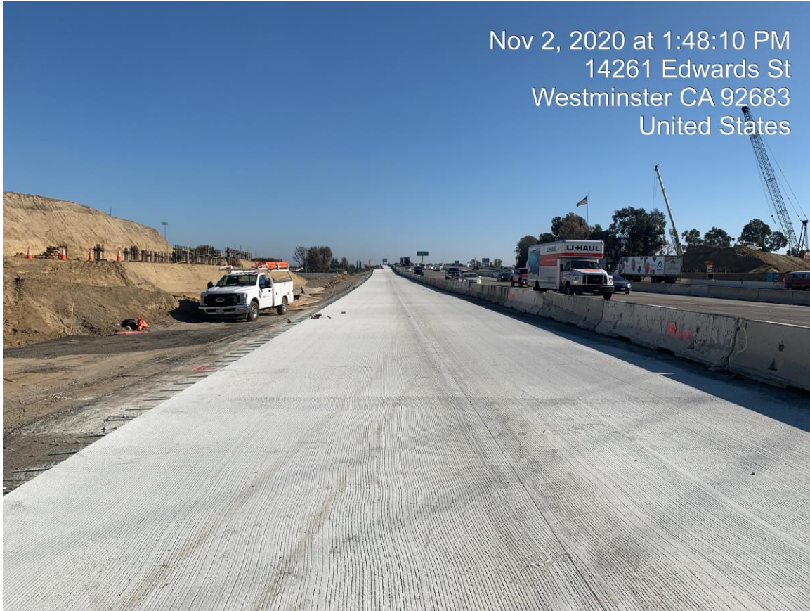
Concrete paving
