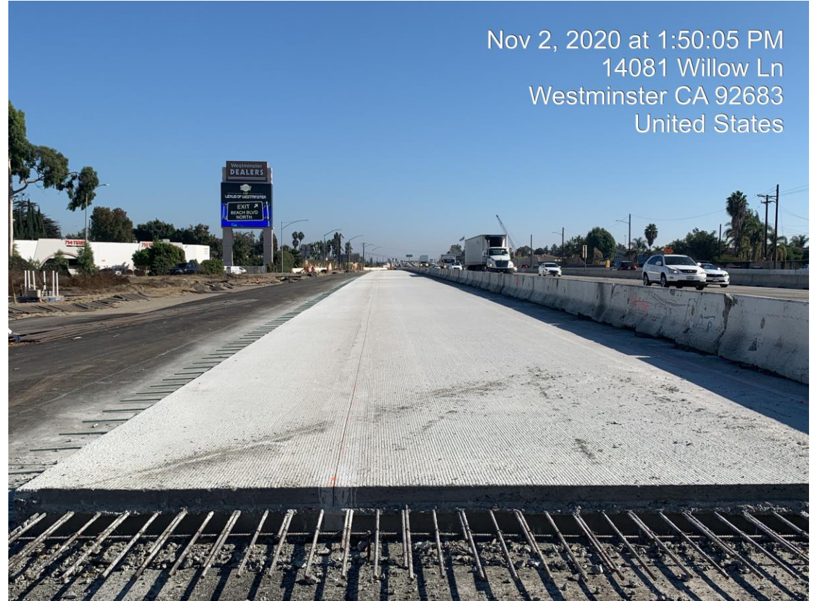
Concrete paving
