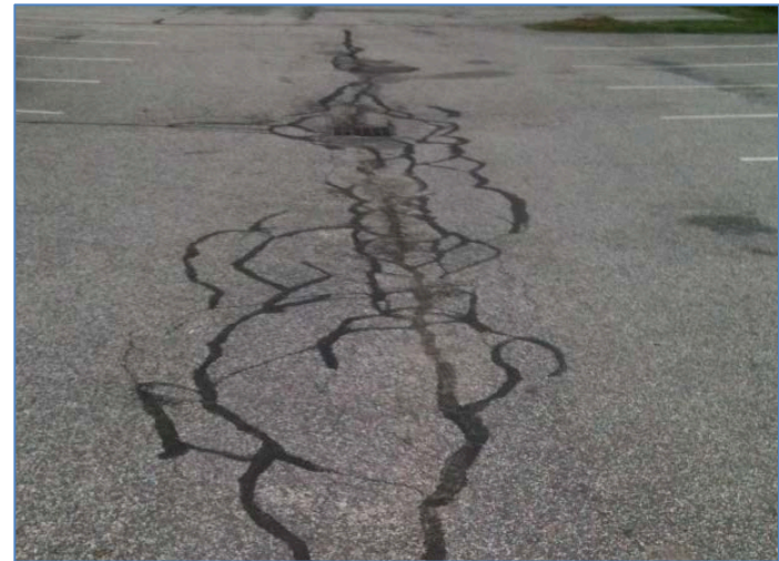
Crack Seal
