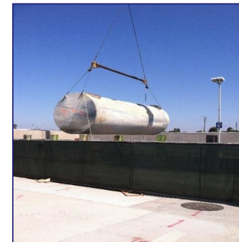
Underground Diesel Tank Removals Anaheim Base
