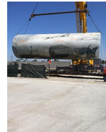
Underground Diesel Tank Removals Anaheim Base
