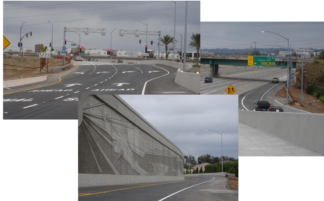
Westbound 91 auxiliary lane from SR-55 and Tustin Avenue off-ramp improvements
