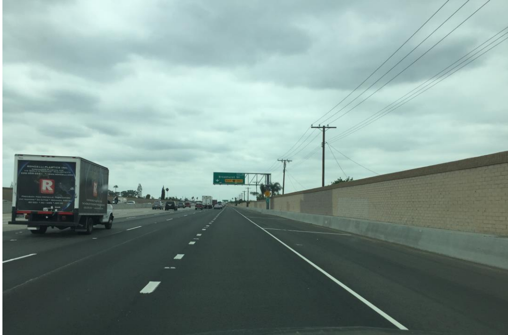
Westbound 91 lane addition from SR-57 to I-5
