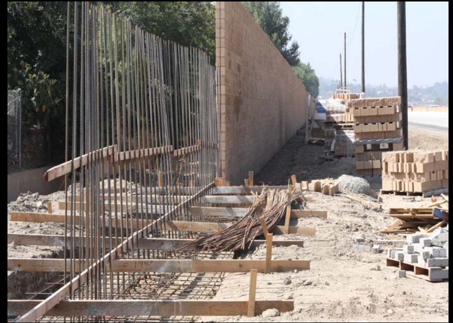
Rebar, foundation, and block work
