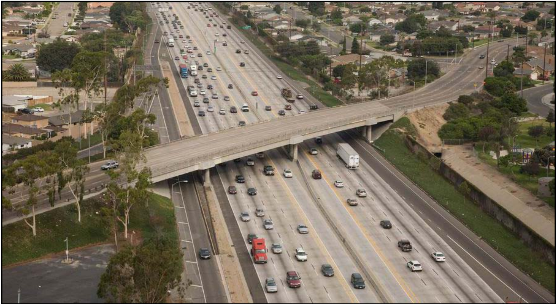
I-405 looking northwest at Springdale Street overcrossing
