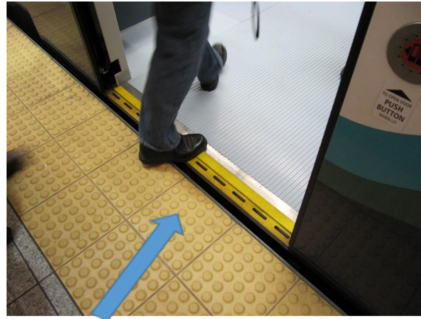
Fully-level Boarding - No bridge plate, ramp or step
