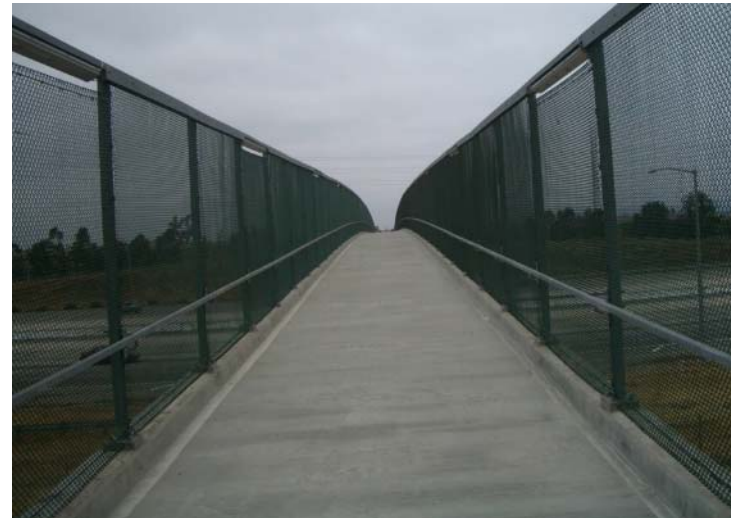
Jeffrey Open Space Trail with existing bridge over I-405
