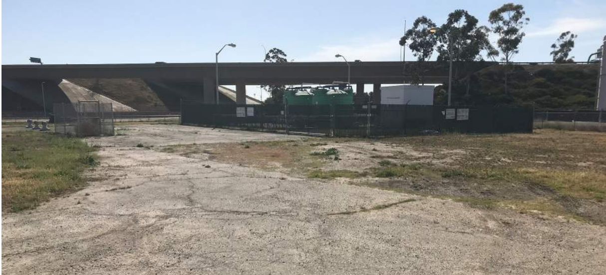
PHOTO 6: EXISTING PUMP HOUSE COMPOUND NORTHWEST OF THE PROJECT PROPERTY
