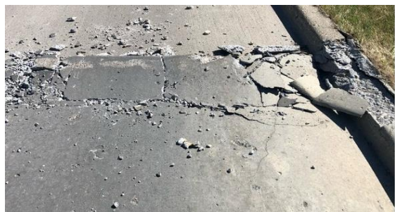
Figure 4-3. Road Buckling 26
