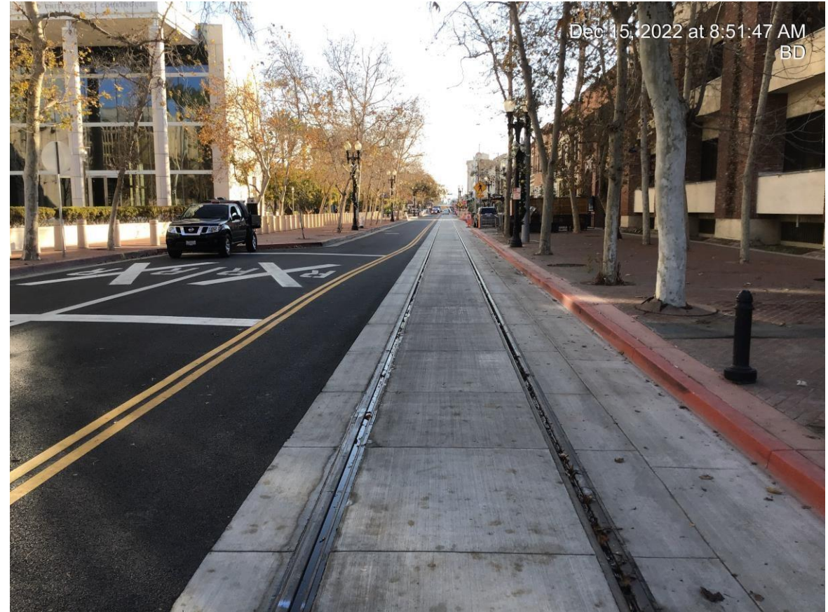
Between Broadway and Ross Street
