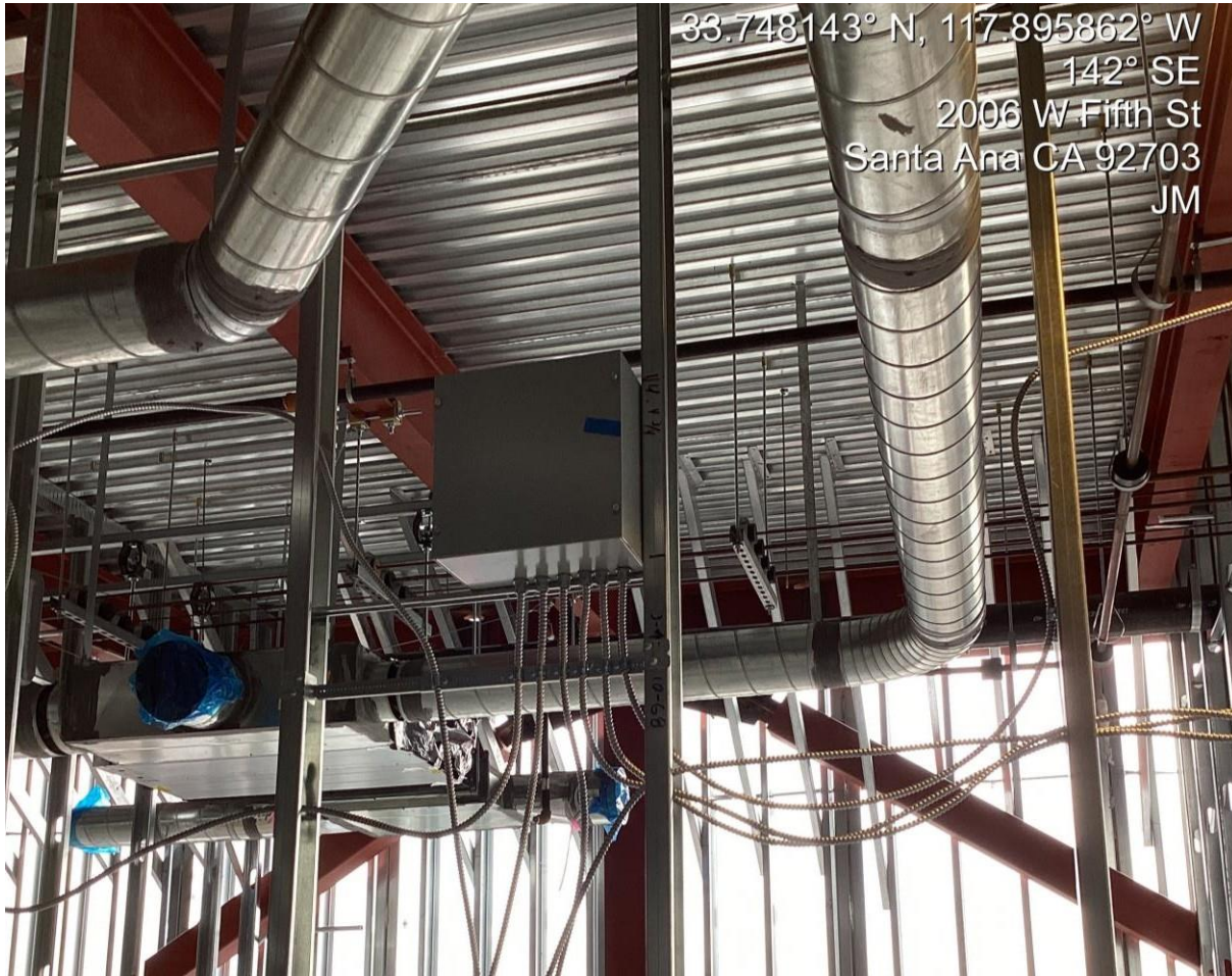
Interior Walls, Piping and Heating, Ventilation, and Air Conditioning
