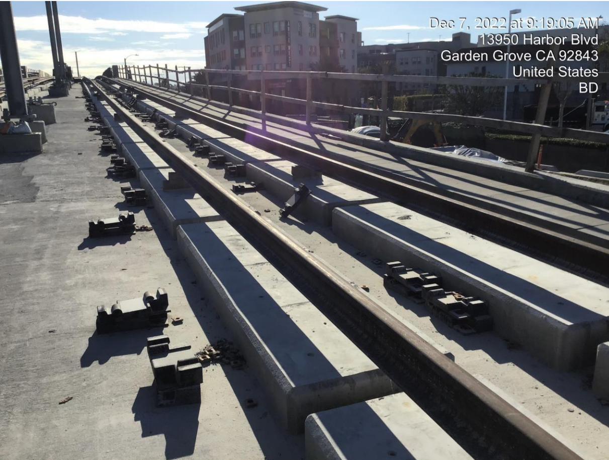
Westminster Bridge Plinths
