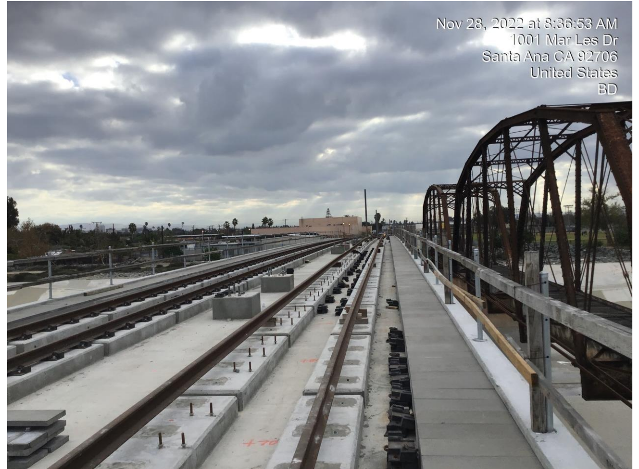
Santa Ana River Bridge Plinths
